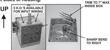
1. Install standard 4" x 4" x 2 1/8" DEEP J-box, together with 1 1/2" extension ring. AC power input wiring can be routed through 5 KO locations in lower J-Box, as shown above. TRIM AC INPUT WIRING TO LENGTH AND SHAPE AS SHOWN
