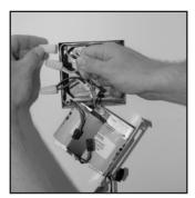
2. Make AC wiring connections to Base Plate Assembly with standard wire nuts. BLACK: 120/277 VAC Universal Input WHITE: NEUTRAL
