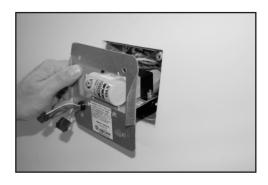
3. Connect polarized battery plug and install Base Plate Assembly into J-Box. Route AC wiring and wire nuts into space above battery.
